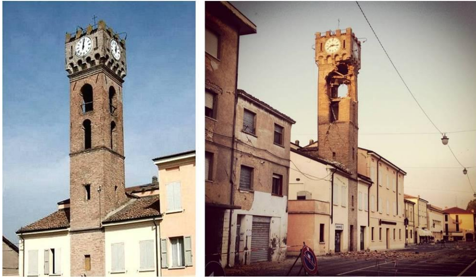
Fig. 2.9 Collapse of the Bell Tower of Novi (Modena), Before the earthquake (left) and after (right)
