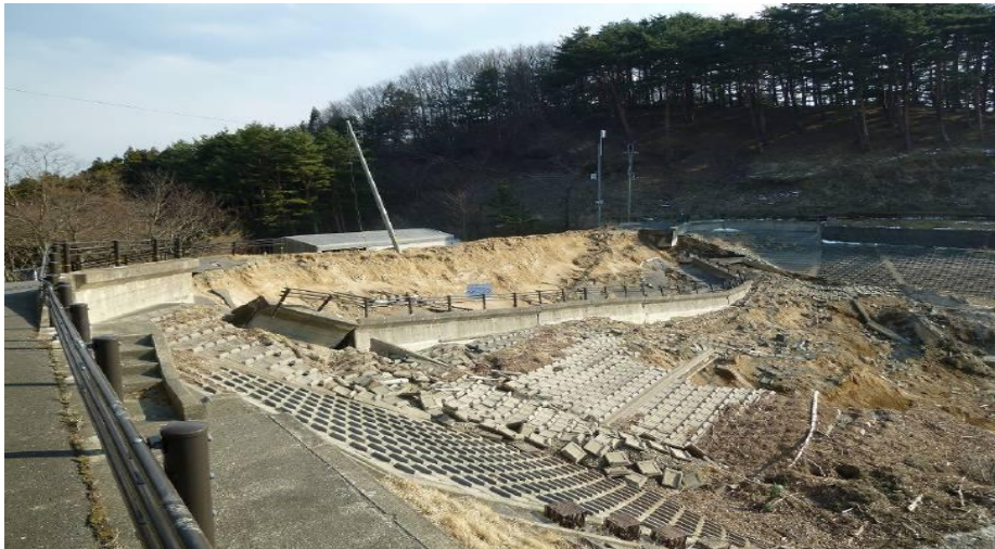
Fig. 2.4 Collapse of Fujinuma dam, Japan 2011
