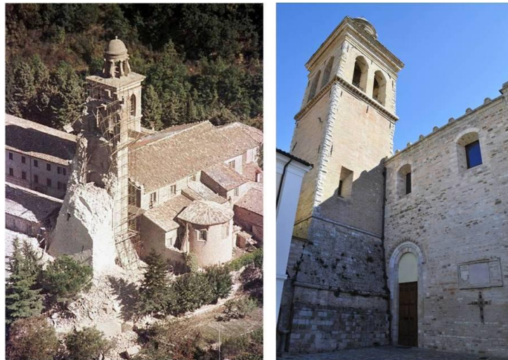
Fig. 2.6 Bell Tower of Nocera Umbra cathedral: after collapse (left) after reconstruction (right)
