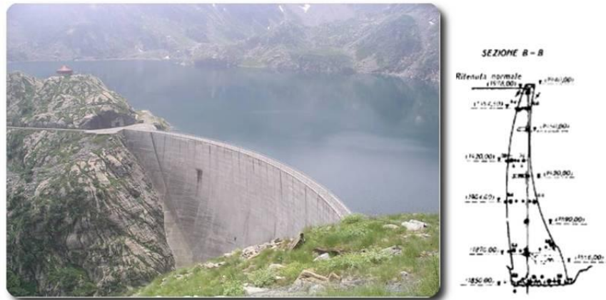
Fig. 5.6 Example of arch-gravity dam
