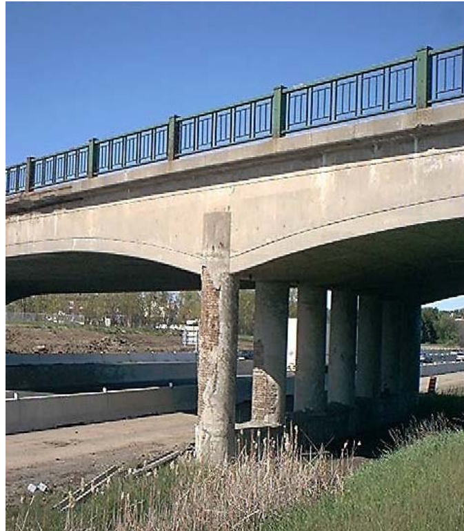
Figure 7.1 Corrosion of rebar in the highway bridge: a) corrosion of the pier b) corrosion of the rebar and spalling of the cover concrete of the wall c) overview of the highway bridge (Tullmin, 2010)
