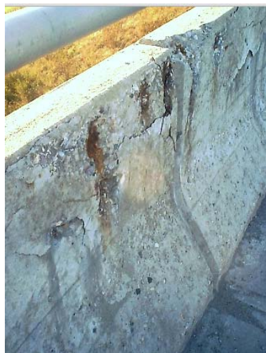
Figure 7.6 Stage 4 of corrosion (Tullmin, 2010)
