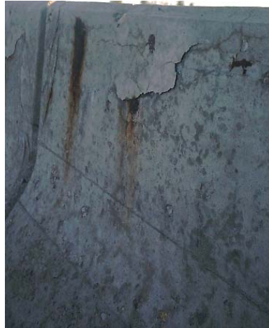
Figure 7.5 Stage 3 of corrosion (Tullmin, 2010)
