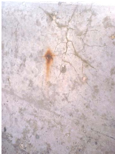
Figure 7.4 Stage 2 of corrosion (Tullmin, 2010)
