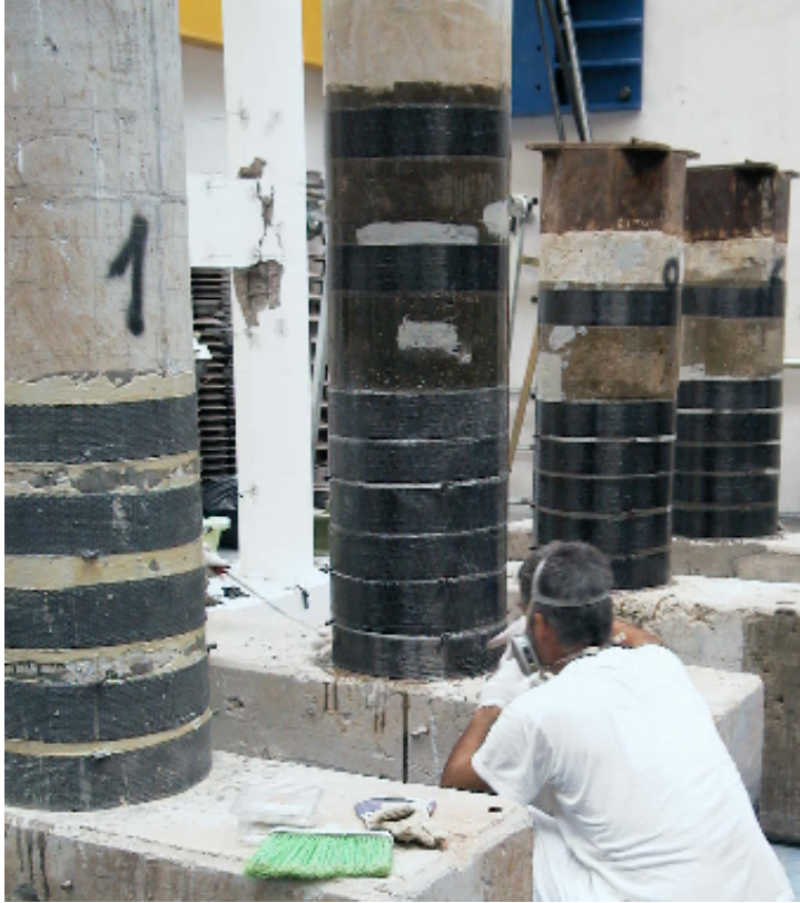
Figure 24 FRP strips application. Tall and squat piers.
