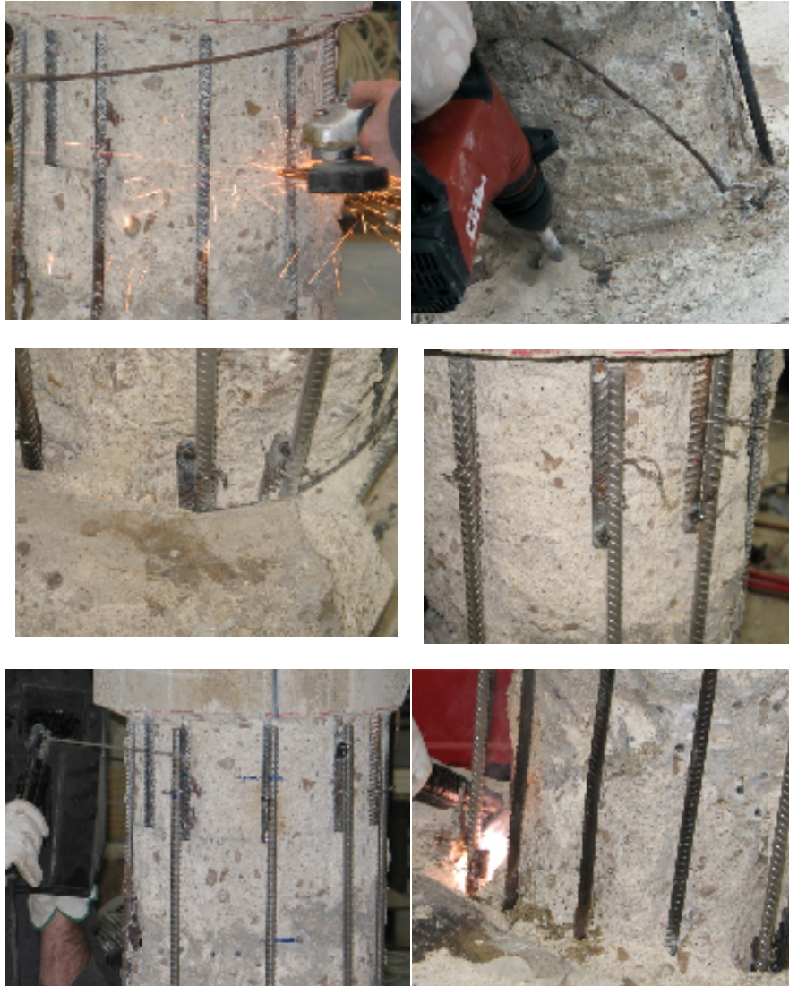
Figure 15 Longitudinal Reinforcing bar restoration (phase 3).(Pier 6)
