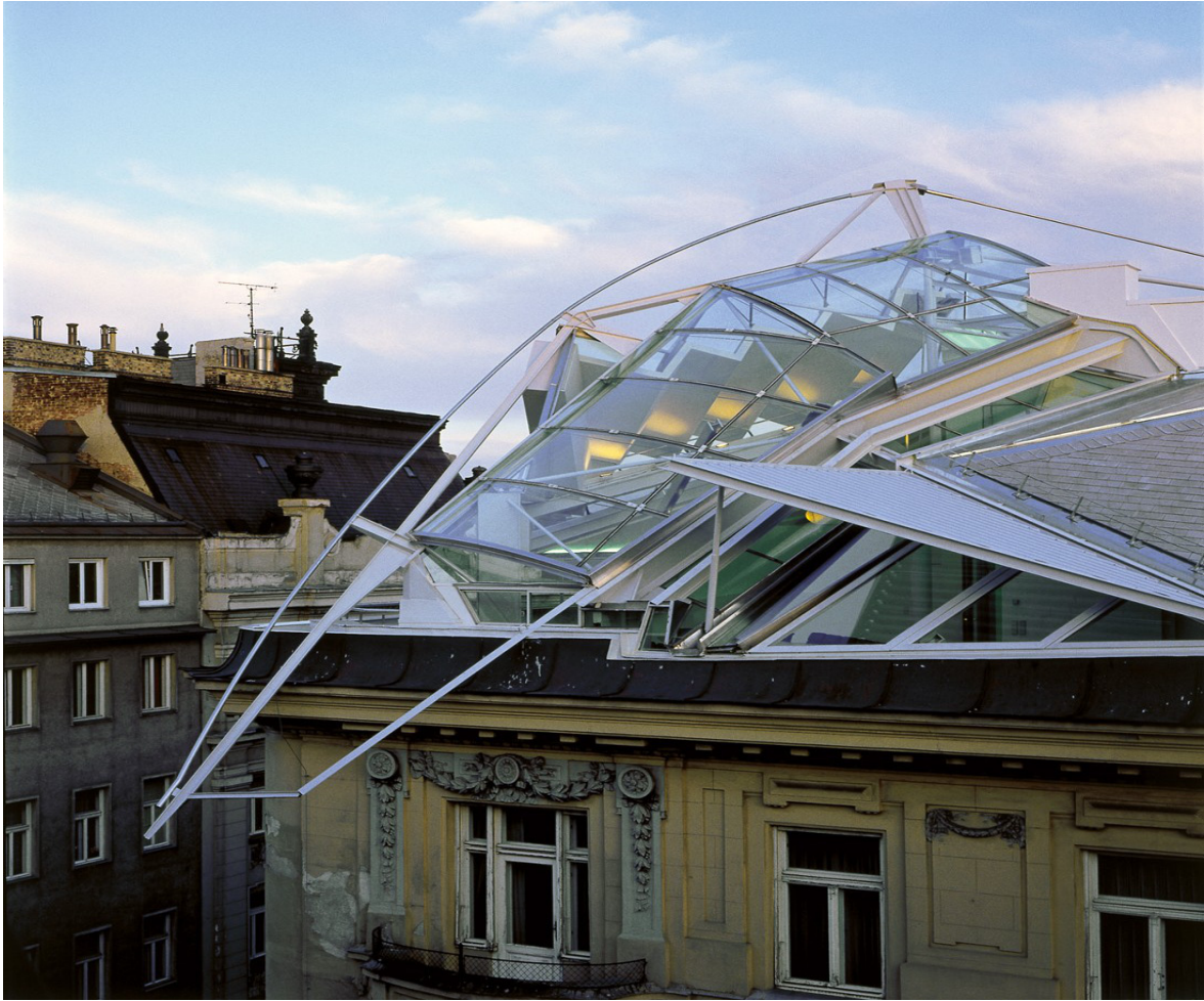
Rooftop Remodeling Falkestrasse , Coop Himmelb(l)au.
