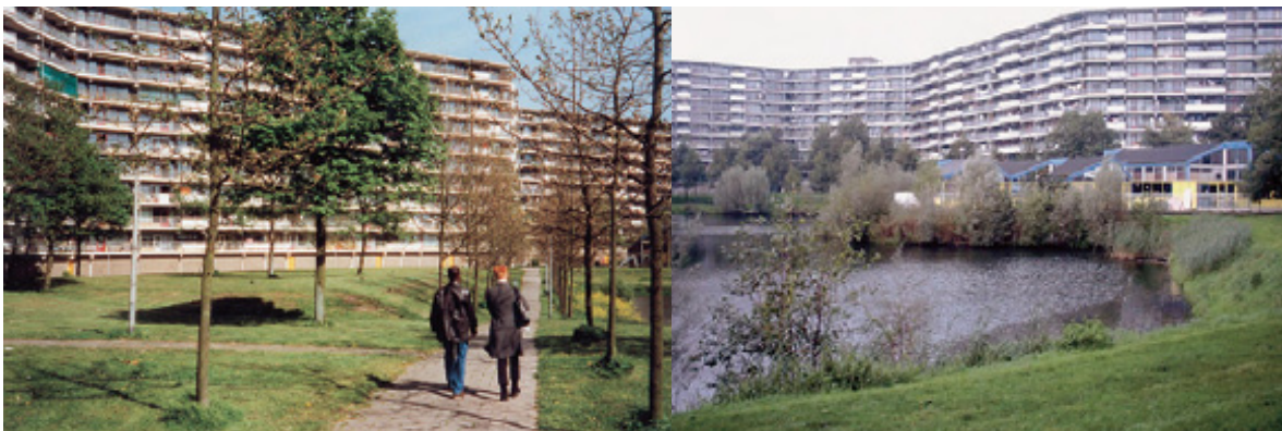
Il Bijlmermeer. (fonte: Wassenberg F. (2006) “The integrated renewal of Amsterdam’s Bijlmermeer high-rise”, in Informationen zur Raumentwicklung.)
