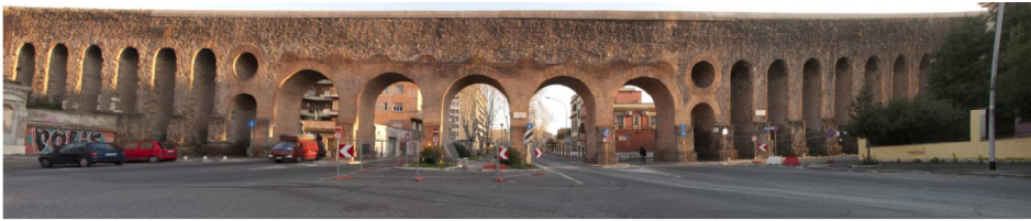
Figure 5.31 View of the Felice aqueduct in the area of Lodi square. Low span arches are the originals ones built with tuff masonry in XVI century while large span arches were built in 1930 with solid brick masonry, Sebastianelli (2011).
