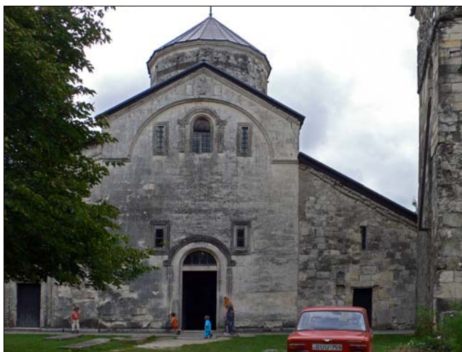
Fig. 1 - The entrance of the church in correspondence with the western porch
