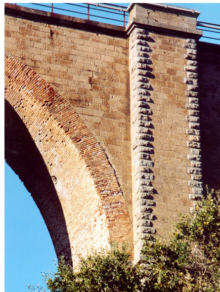
Figure 4.17. Ordinary piers and piers with buttresses.
