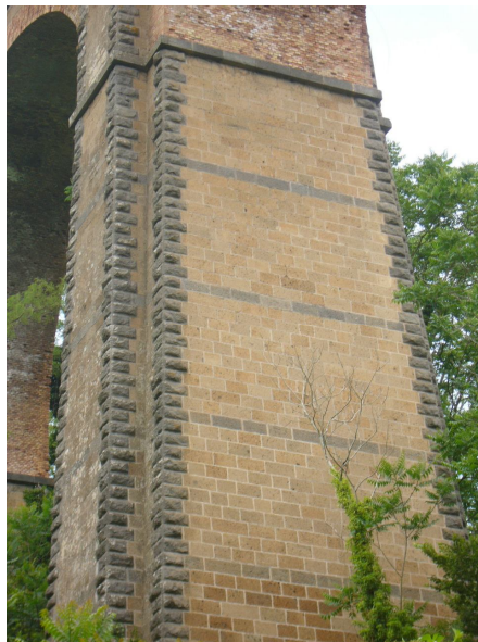
Figure 4.17. Ordinary piers and piers with buttresses.
