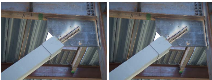
Figure 4.6 Connection to steel structure
