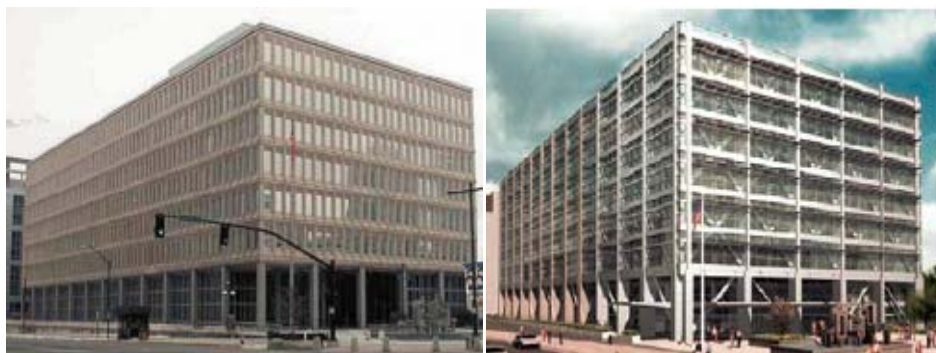
Figure 4.2 retrofitting existing building with dissipative braces
