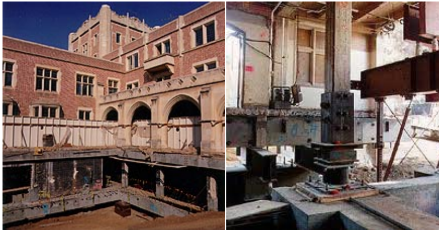
Figure 4.1 retrofitting existing building with base isolation
