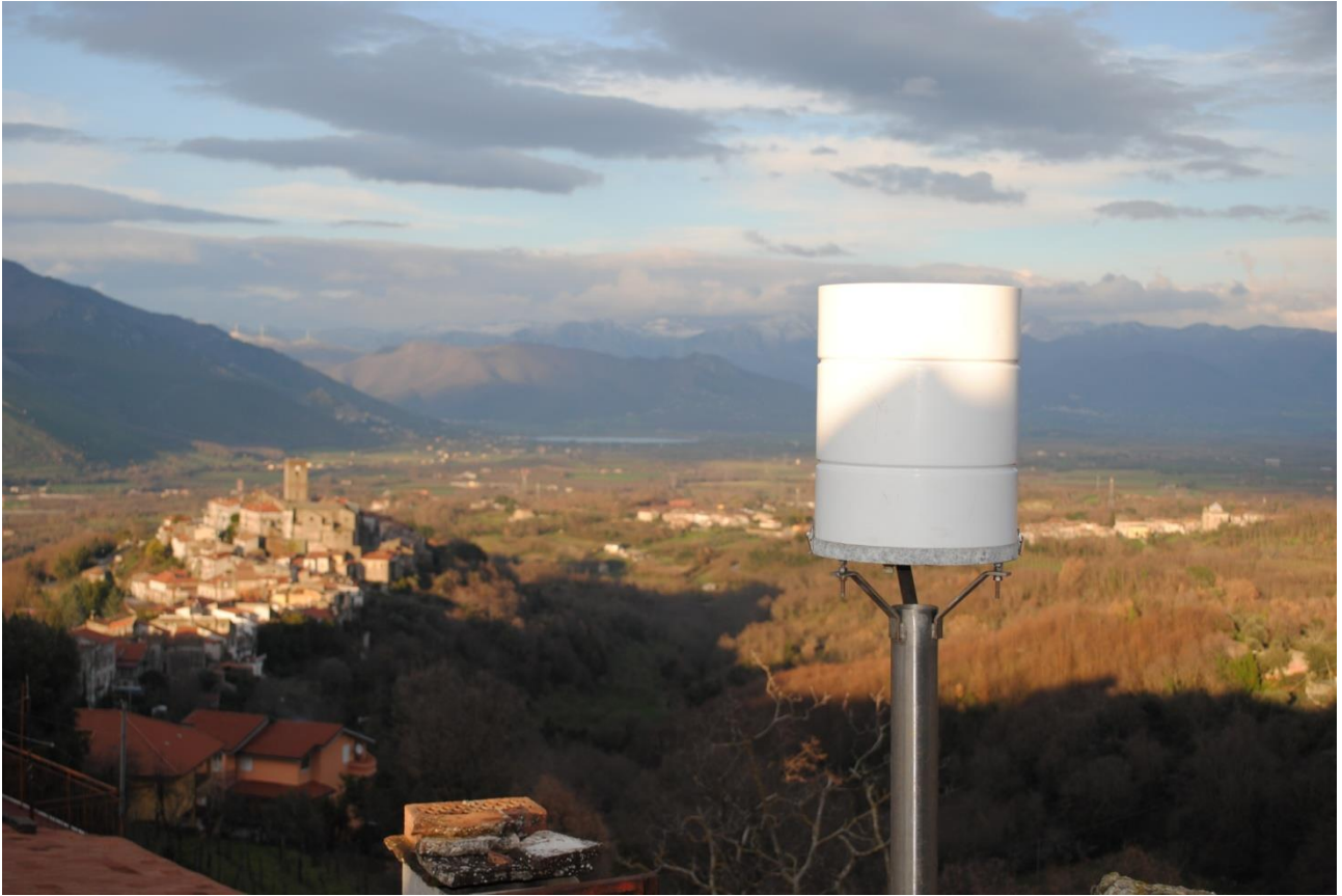
Figure 24 Rain gauge installed in Tora Town
