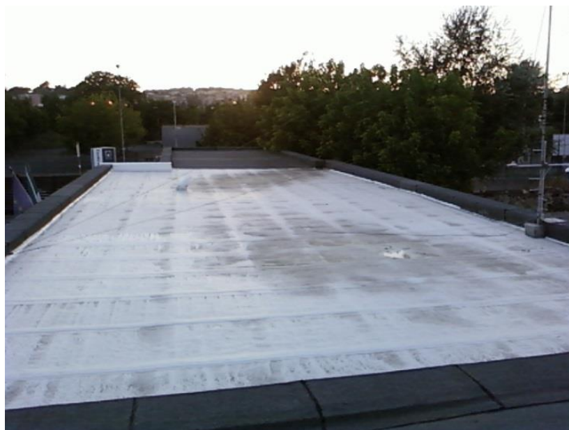
Figure 4.6: Dust and soil effects on mineral membrane.
