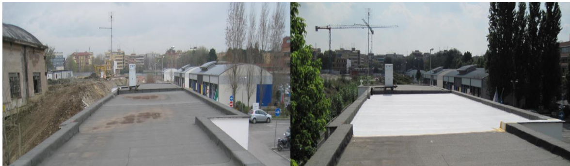
Figure 4.3: Roof before and after the application of the reflective membrane.
