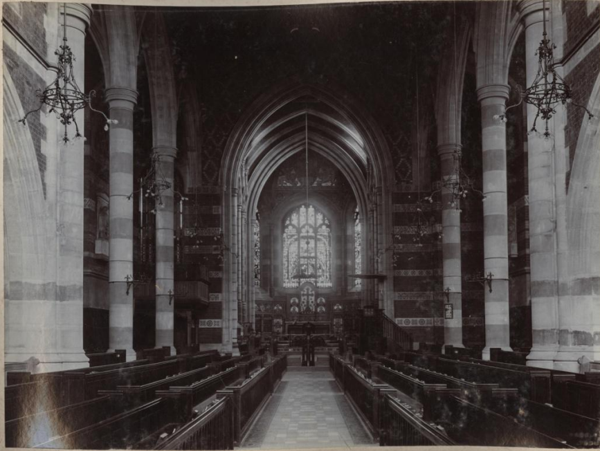
Interior of chapel (looking east)
