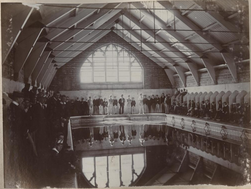
Interior of school bath.
