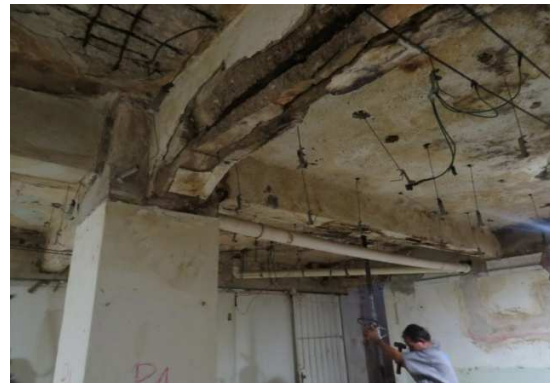
Figure 3.10 Extreme case of deterioration of the Ouro Branco building, built in 1935, in the center of São Paulo. Steel corrosion and concrete spalling caused by carbonation of concrete, with cross-section loss of reinforcement (photographs taken in January 2014)
