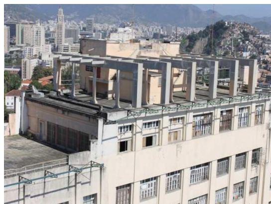
Figure 2.17 Current photo of the building's roof, taken in July 2014
