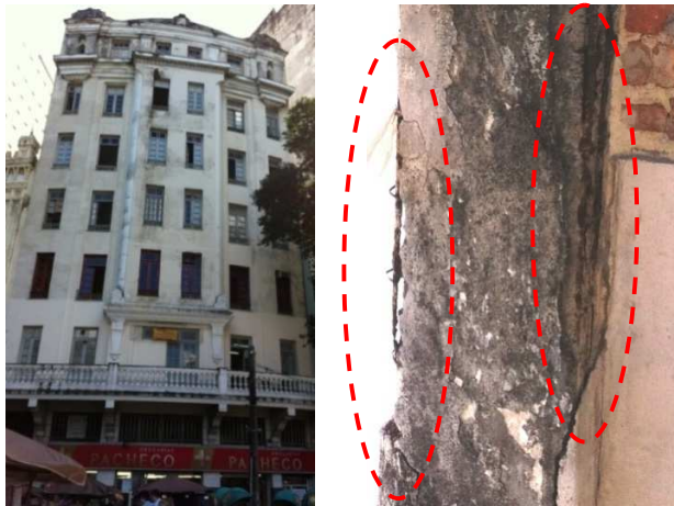
Figure 3.06 Deterioration of the slab of the 1st floor. Reinforcement corrosion and concrete spalling likely caused by chloride attack. Heritage building belonging to Monastery of São Bento , located in marine environment, in the center of Rio de Janeiro (photographs taken in July 2014)
