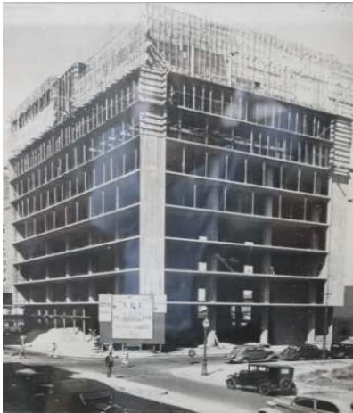
Figure 2.24 ABI Building during construction
