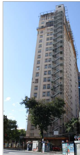
Figure 7.02 Lateral façade of the building (photo taken in July 2014)
