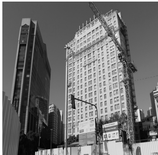
Figure 2.22 Building photograph taken in July 2014
