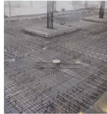
Figure 2.44 Photographs of the slab reinforcements, taken in 1939. On the right, reinforcement of the capitals and on the left, the reinforcement of the merged beams in the slab
