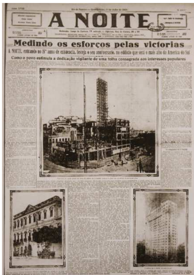
Figure 2.08 Brazilian newspapers called A Noite of July 18, 1928, with some photos of the construction of the A Noite building
