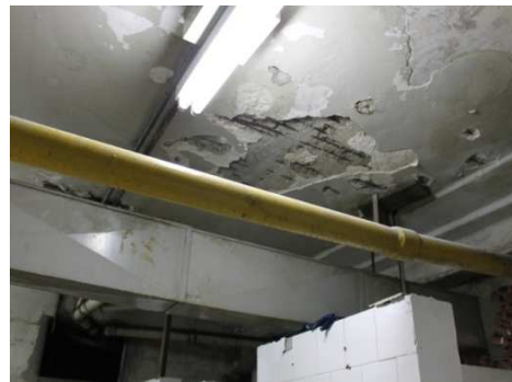
Figure 3.09 Structural deterioration of the ground floor and roof floor. Concrete spalling and steel corrosion with cross-section loss of the transverse and longitudinal reinforcement, likely caused by chloride attack. A Noite building, built in 1929, located in the marine environment, in the center of Rio de Janeiro (photographs taken in July 2014)
