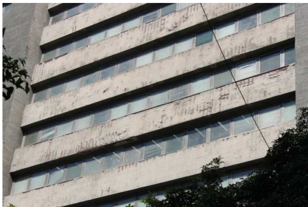
Figure 3.08 Steel corrosion and concrete spalling of columns and beams likely caused by carbonation of concrete (most likely occasioned by having a small layer of concrete cover for reinforcement). Rua Nilo Peçanha building, built in the 50s in the center of Rio de Janeiro (photographs taken in July 2014)
