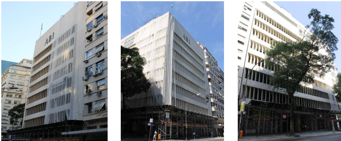
Figure 2.28 Photographs taken in July 2014, during the restoration works of the façades
