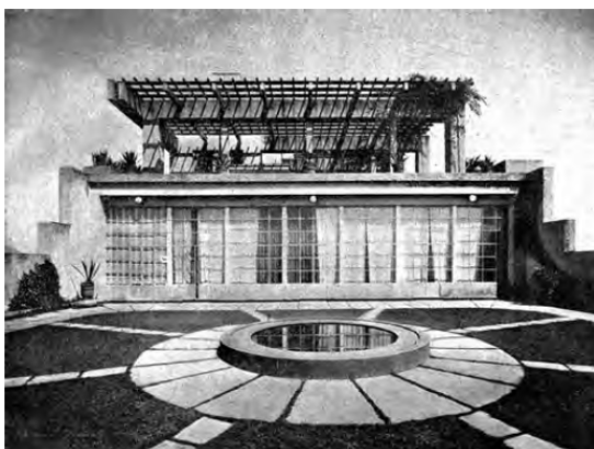
Figure 2.16 View of the pergola after completion of the structural reinforcement works. [Concrete Magazine n. 75 June 1945]:183
