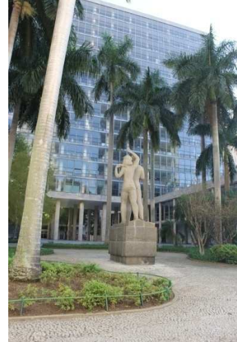
Figure 2.32 Glass façade. Photograph taken in July 2014
