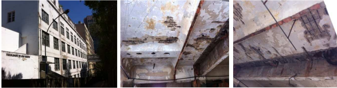
Figure 3.06 Deterioration of the slab of the 1st floor. Reinforcement corrosion and concrete spalling likely caused by chloride attack. Heritage building belonging to Monastery of São Bento , located in marine environment, in the center of Rio de Janeiro (photographs taken in July 2014)
