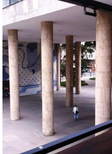
Figure 2.31 Double Pilotis . Photograph taken in July 2014
