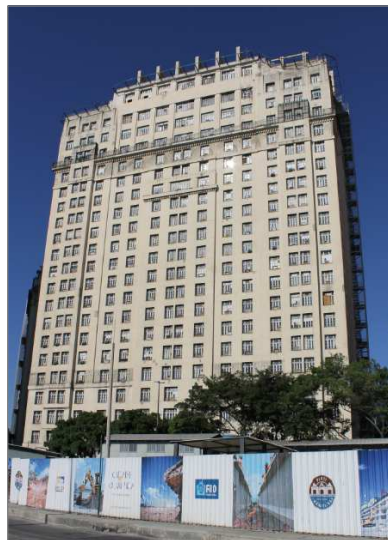
Figure 7.01 Front façade of the building (photo taken in July 2014)
