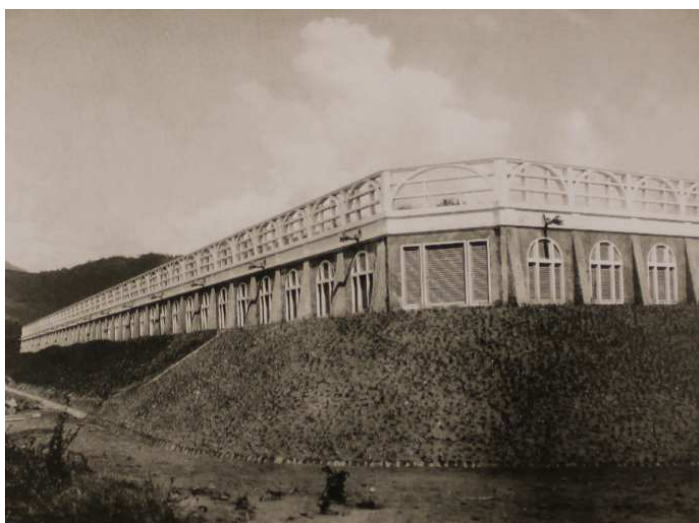
Figure 2.02 Water reservoir of the Engenho de Dentro (built in reinforced concrete, circa 1908)
