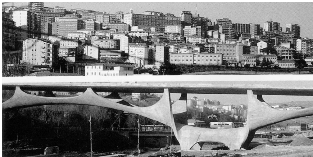
Figure 4.3: Front view of the Basento bridge [Image in the public domain]
