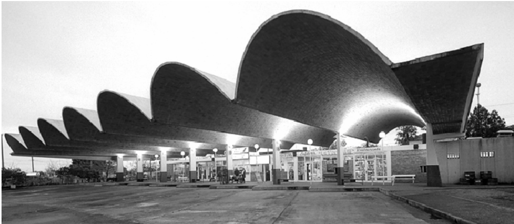
Figure 2.13: Municipal bus terminal in Salto by Eladio Dieste (Uruguay, 1974) [PC: Vicente del Amo]
