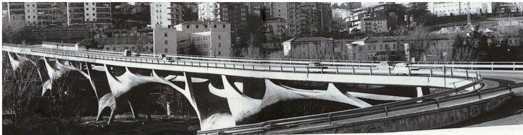
Figure 4.2: View of the Basento bridge [Image in the public domain]
