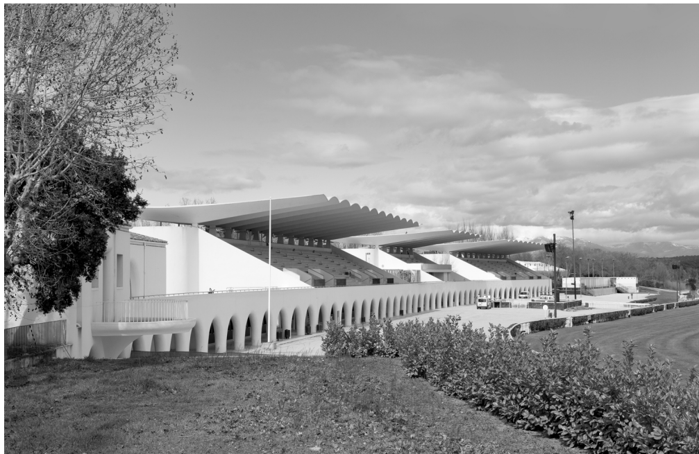
Figure 2.17: Zarzuela's Hippodrome by Carlos Arniches Moltó, Martín Domínguez Esteban and Eduardo Torroja (Madrid, 1941) [PC: Ana Amado]
