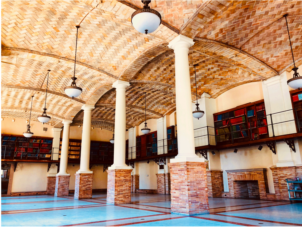
Figure 2.12: Guastavino Room in the Boston Public Library by Rafael Guastavino (Boston, 1895) [PC: Author]
