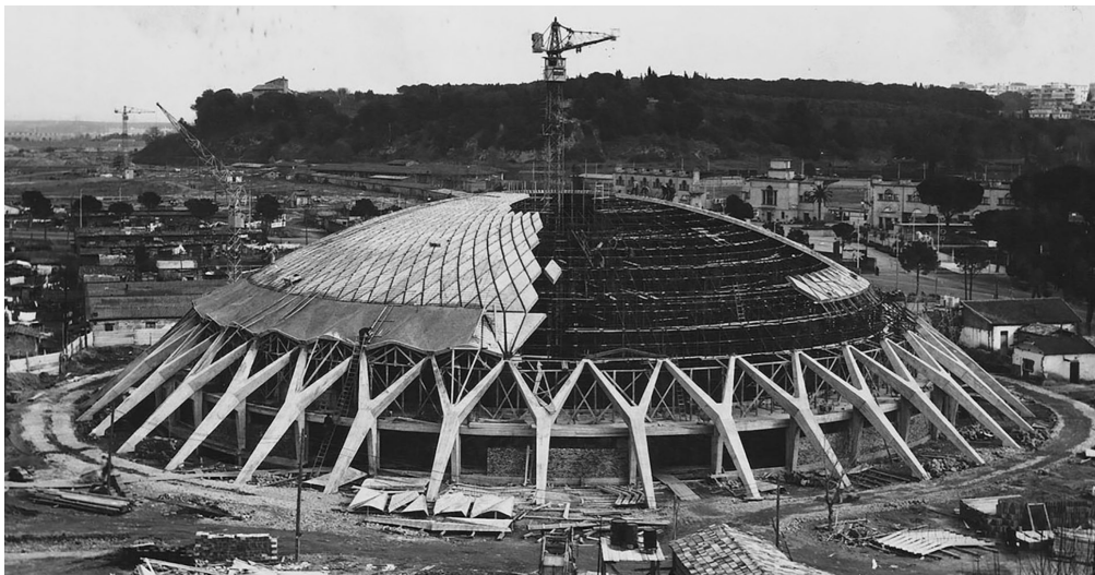
Figure 2.15: Palazzetto dello Sport by Annibale Vitellozzi and Pier Luigi Nervi (Rome, 1957) [Image in the public domain]
