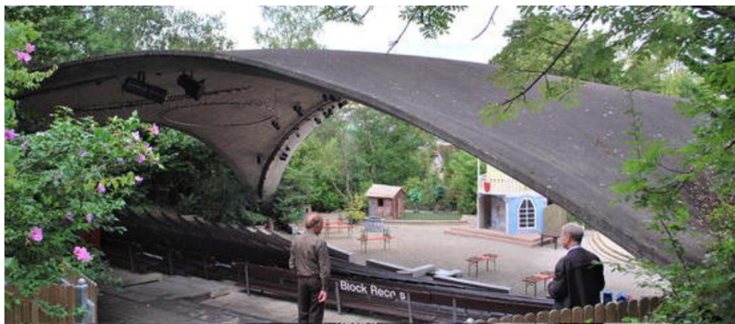
(c) Form-found: Open Air Theatre in Grötzingen by Heinz Isler (Germany, 1977) [PC: John Chilton]
