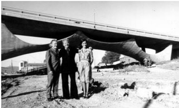
Figure 4.1: Sergio Musmeci (left) in front of the Basento bridge [PC: Paolo Musmeci]
