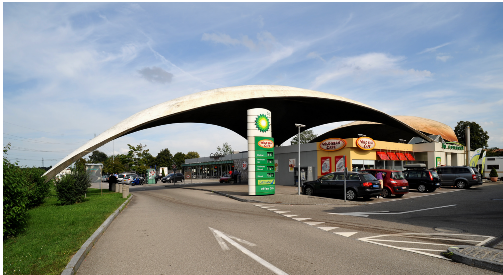
Figure 3.9: Motorway service station in Deitingen by Heinz Isler (Switzerland, 1968) [via wikimedia.org]
