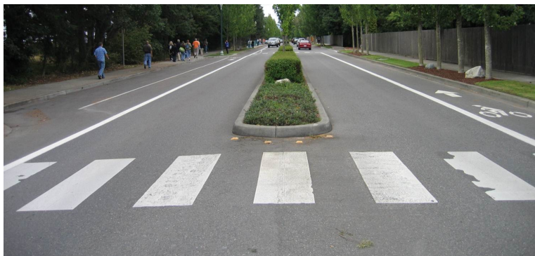
Figure 3.5: Example of raised island at bicycle crossroad.
