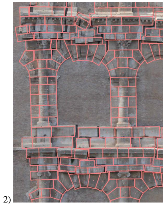
Figure 4.26 Matching of the existing and pulse-by failure patterns
