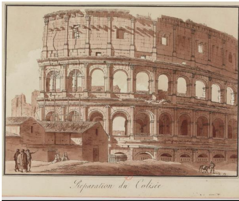
Figure 4.10 Timber shoring in the south-east wall in 1806-1807 (Uggeri 1809)
