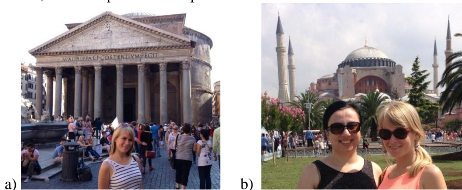
Figure 2.2 Examples of the great masonry dome structures: a) Pantheon, Rome and b) Hagia Sophia, Istanbul
