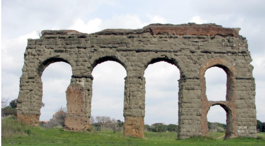
Figure 5.3 Example of the ancient retrofitting brick works
