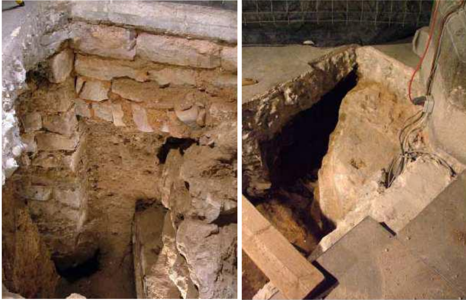
Figure 4.23 Butters (left) and piers (right) foundation.
