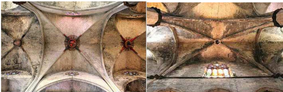
Figure 4.20 Square and rectangular cross vaults of the central (left) and lateral (right) nave of Santa Maria del Mar.
