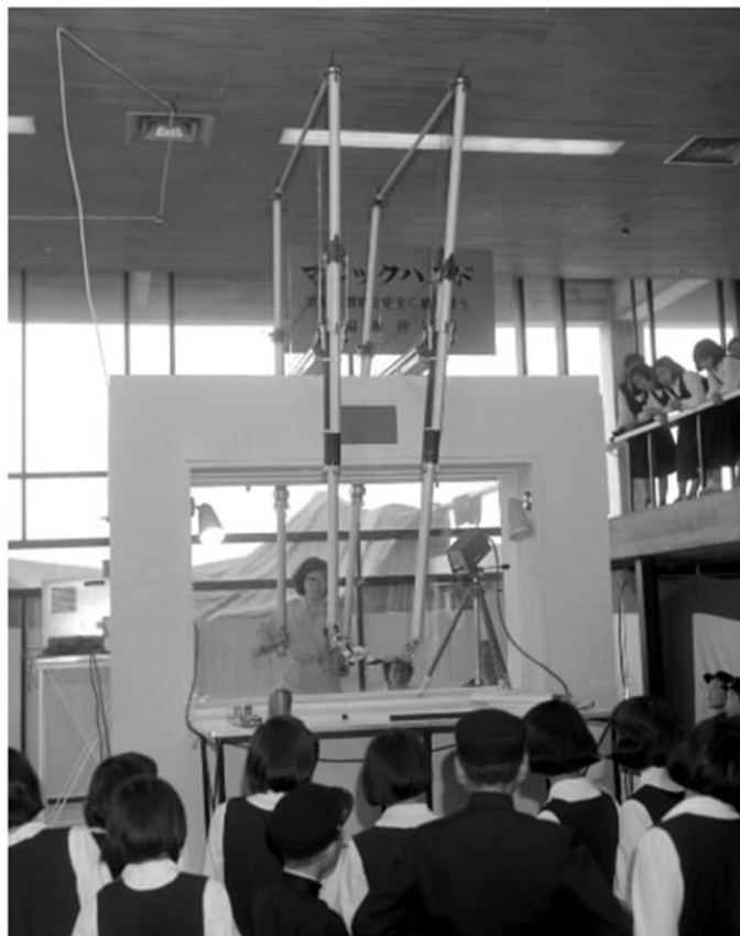
Schoolchildren watching a demonstration of “The Magic Hand,” Hiroshima ‘Atoms for Peace’ Exhibit, November 1956. “The Magic Hand,” designed for the remote handling of radioactive material, was used at the exhibit to pour liquid from a bottle to a cup, or for calligraphy with a brush. (source: Archives of Hiroshima City)
