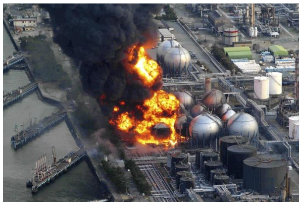
Figure 2.3. LPG tanks burned at the Cosmo oil refinery in Ichihara city, Chiba Prefecture after the 2011 Tōhoku earthquake (Reuter 2011)
