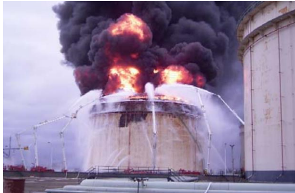
Figure 2.2. Full-surface fire of naphtha tanks occurred after two days of the 2003 Tokachi-oki earthquake (Hatayama et al. 2008)
