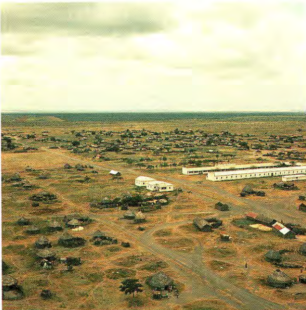
28) Aerial view of parts of the failed nomadic agricultural resettlement scheme of Sablaale on the Shabeelle river (Janzen, 1984).
