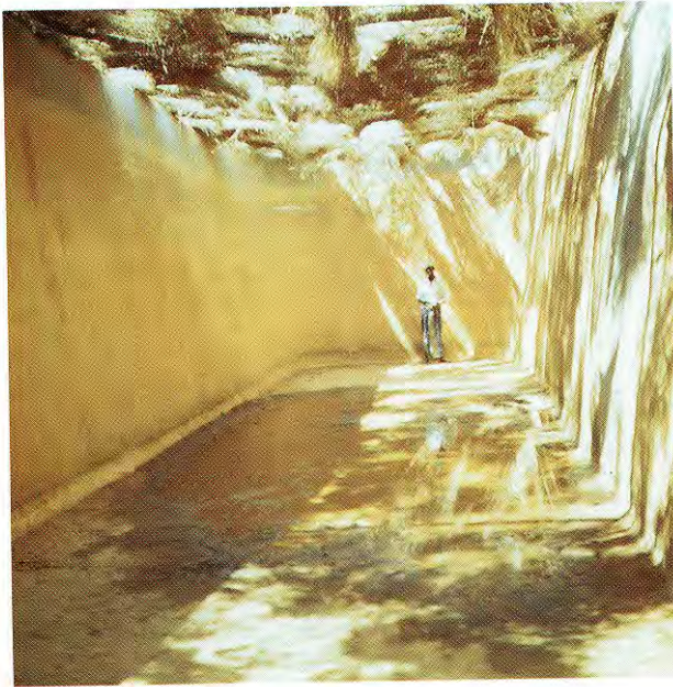
24) As a result of an increasing commercialisation the nomads could afford to construct water catchments ( sing.: berked ) throughout arid central and northern Somalia (Janzen, 1982).
